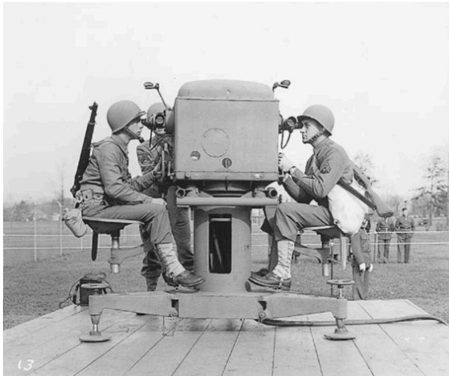
Fig. 9.1. M-9 gun director, tracking head with operators. One follows the target in elevation, the other in azimuth. The unit and the operators rotate while tracking. Courtesy of AT&T Archives.
